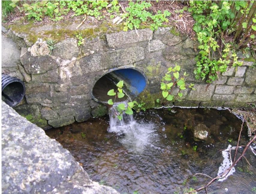
Fig. 1.3 Penetration of mortared joints of a bridge structure GR SW 3728 3181
