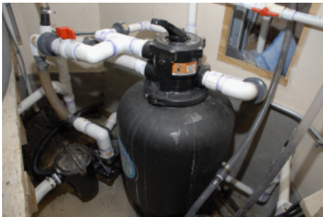
Plate 2. A simple rapid sand filter designed for whirlpool baths and small swimming pools is excellent for filtering larger volumes of water. These are readily available from many sources. R. A. Odum, Toledo Zoological Society.
