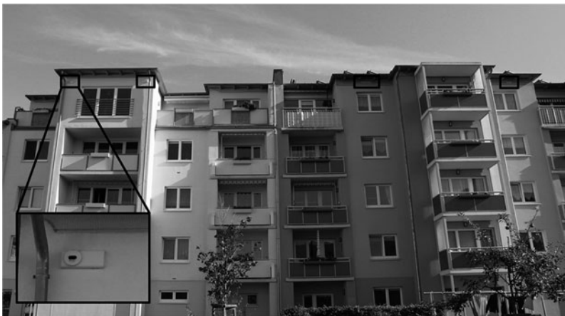
Figure 1. A section of a renovated prefabricated apartment-complex in Greifswald with five compensatory nest-boxes for Common Swifts (box type Schwegler 17 ). The boxes are integrated in the thermal insulation. Photograph by T. Schaub.
